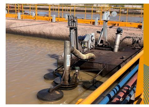
Our customer needed a complete solution adapted to the size of their wastewater basins. Our engineers developed a complete system able to move the Surfcleaner to filter debris and to extract processed oils".
