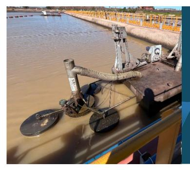
"Our customer from the Steel Processing Industry needed a complete solution adapted to the size of their wastewater basins. Our engineers developed a complete system able to move the SurfCleaner, to filter debris and to extract processed oils."
